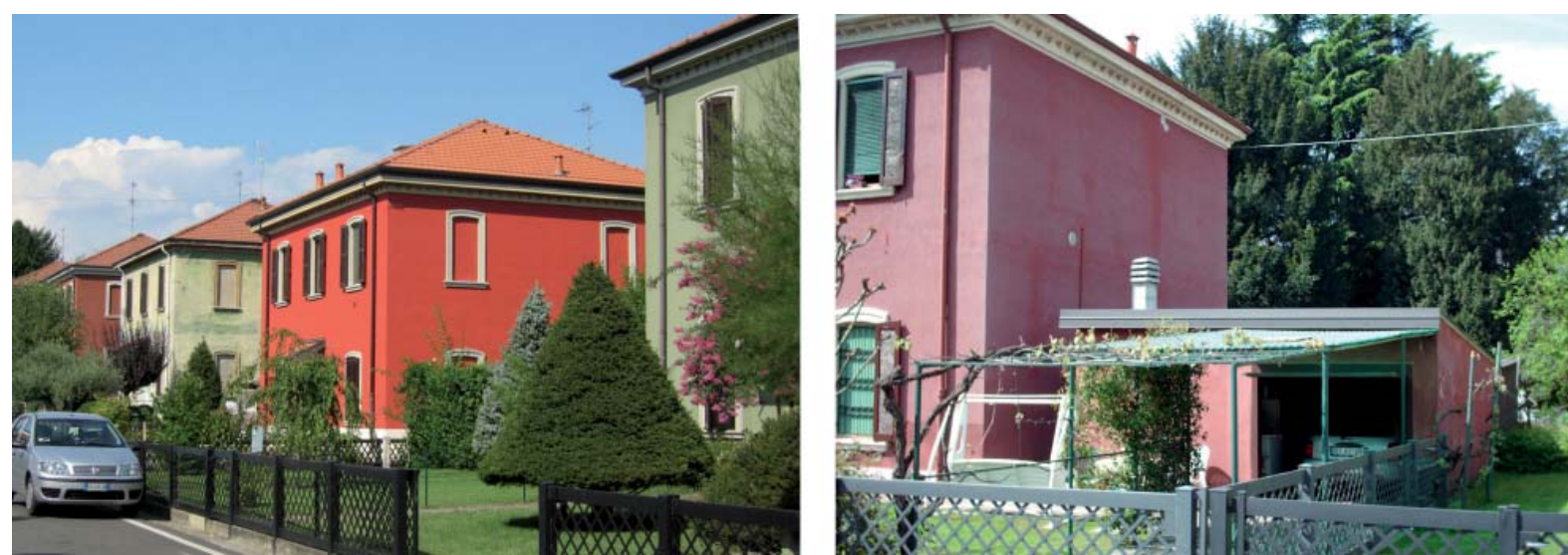
Fig.3 - A recent intervention on external surfaces; Fig.4 - An ancillary structure used as storage and garage
